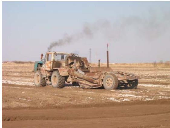
Photo 8. A receiver is mounted on the leveling equipment.
