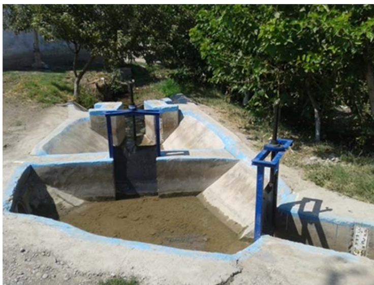
«Kahramon Davlat Sahovati» farm, Experimental field of the SIC-ICWC, facility for water supply and measurement
